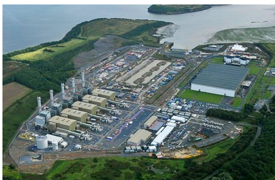
Obr. 44: Pembroke Zdroj: premierconstructionnews.com
